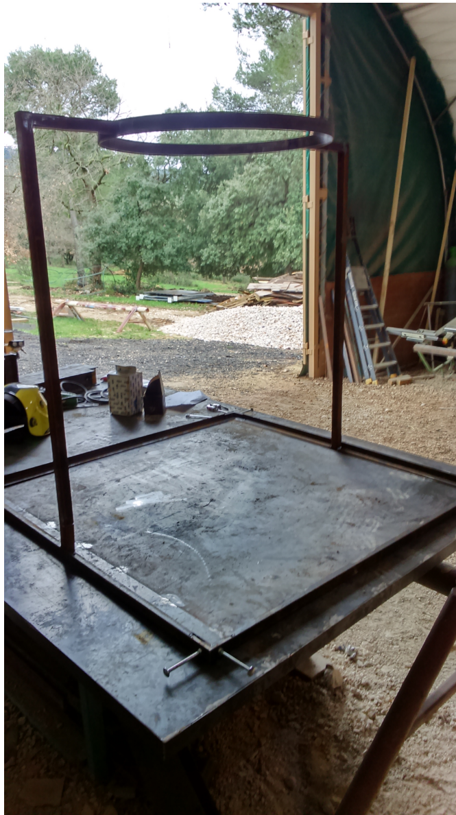
FIGURE 4.42.: 1 er montage du support
